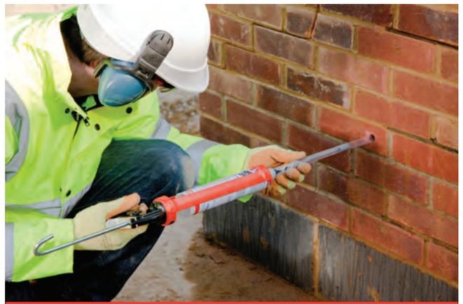
Injecting resin to complete the RetroTie installation
