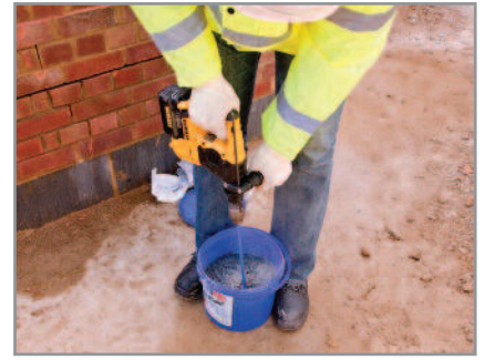
3. Stir thoroughly using a power-driven paddle mixer. Do not attempt to mix by hand as this is likely to lead to erratic results
