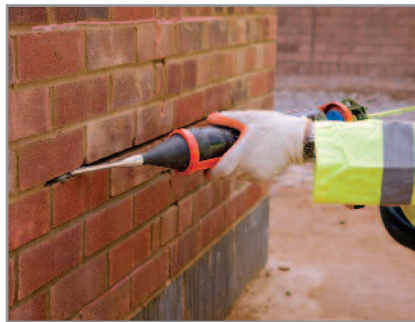
5. Inject into the slot or hole in a continuous operation. Typical working life of the mixture in the pail is around 2 hours with re-agitation . The cartridge should be emptied within 5 minutes. If the injection process is interrupted for any reason, empty any cartridge contents back into the bucket and re-stir until it again reaches a smooth injectable consistency
