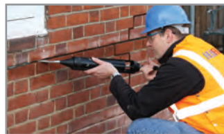
3. Using the Helifix Pointing Gun, inject a bead of HeliBond along the back of the slot
