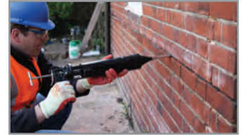
5. Insert a further bead of HeliBond over the exposed HeliBar, finishing 12mm from face and 'iron' firmly into the slot using the HeliBar Insertion Tool
