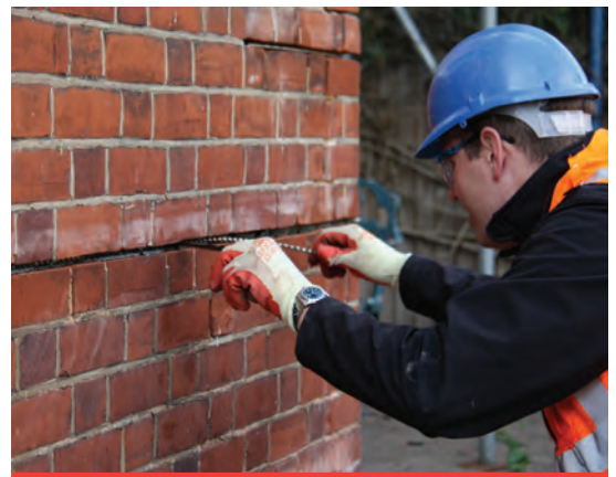
HeliBar is inserted into HeliBond grout within a cut slot
