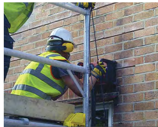
STEP 2 Clean out slots with a blow pump and apply HeliPrimer WB or flush with water.
