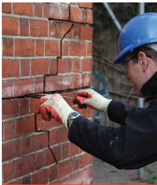
Crack stitching
