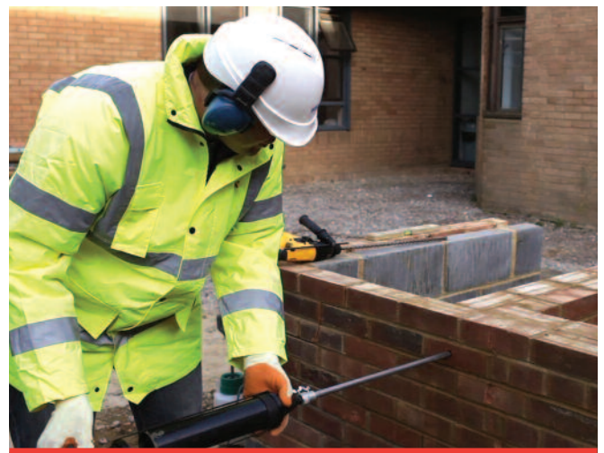
Inserting the grout-filled pinning nozzle, containing the CemTie, into the clearance hole
